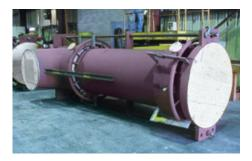
Several **metal expansion joints** are employed in the ethylene cracker at Nova Chemicals in Sarnia Ontario, Canada. Operating conditions: p = 3.45 bar (50 PSI); t = 420 °C (788 °F).
