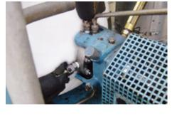
Liquid, high-purity ethylene is pumped in the cracker operated by the Dow Olefinverbund in Böhlen, Germany. The pump shaft is sealed by a **MFLCT80S1** type triple seal. The metal bellows seal has clear benefits at the temperatures down to -100 °C (-148 °F) encountered in this environment. A **TS2000** type Thermosiphon system supplies the seal.
