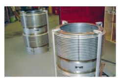
The El Dorado Chemical Co. in Arkansas, USA, uses **metal expansion joints** in the plant for manufacturing nitric acid. Operating conditions: p = 10 bar (145 PSI); t = 649 °C (1,200 °F).
