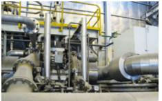
A type **DGS30** gas-lubricated mechanical seal is used to seal a compressor in BASF's synthesis gas plant in Shanghai, China. Nitrogen-buffered **Espey WD400** floating ring seals seal the bearings. The process medium is carbon dioxide. Operating conditions:  $p_1$  (dynam.) = 18.5 bar (268 PSI); t = 70 °C (158 °F); n = 25,750 min<sup>-1</sup>.
