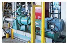
Sealing of a centrifugal pump for the manufacture of aromatic compounds at Shell in the Netherlands. The high drive power of 75 kW makes it necessary to apply a high efficiency **NMB-22P-9R-35-ND** magnet coupling. This uniquely efficient magnetic coupling drastically reduces power losses and the associated heat generation. Operating conditions: p = 35 bar (508 PSI); t = 20 °C (68 °F); n = 990 min<sup>-1</sup>.
